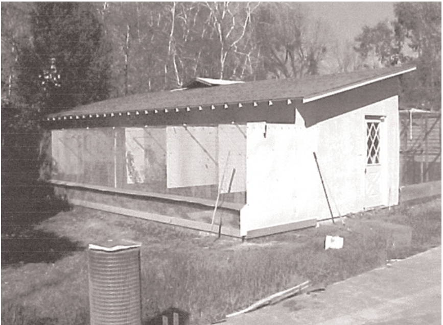
The completed aviary.
