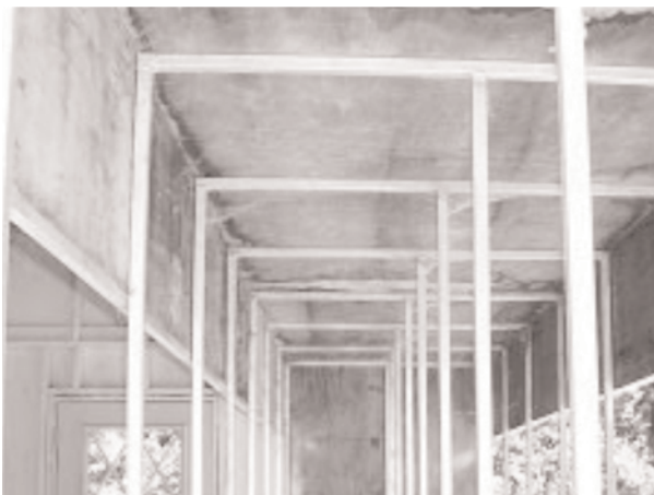
Picture showing steel frame work supporting the ceiling of the flights and above that, the roof.
